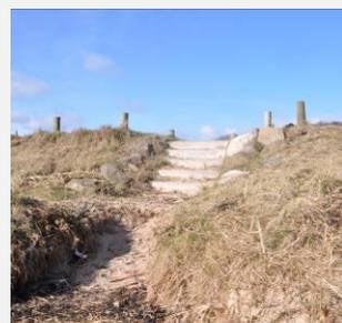
Last year's high autumn tides coincided with strong winds and washed over the bank by the boathouses, flooding both the road and the Large Boathouse. You will notice that the bank has been built up there, with a paved path over it onto the beach for pushchairs and prams, and hopefully the problem is now solved (photo, top right).
